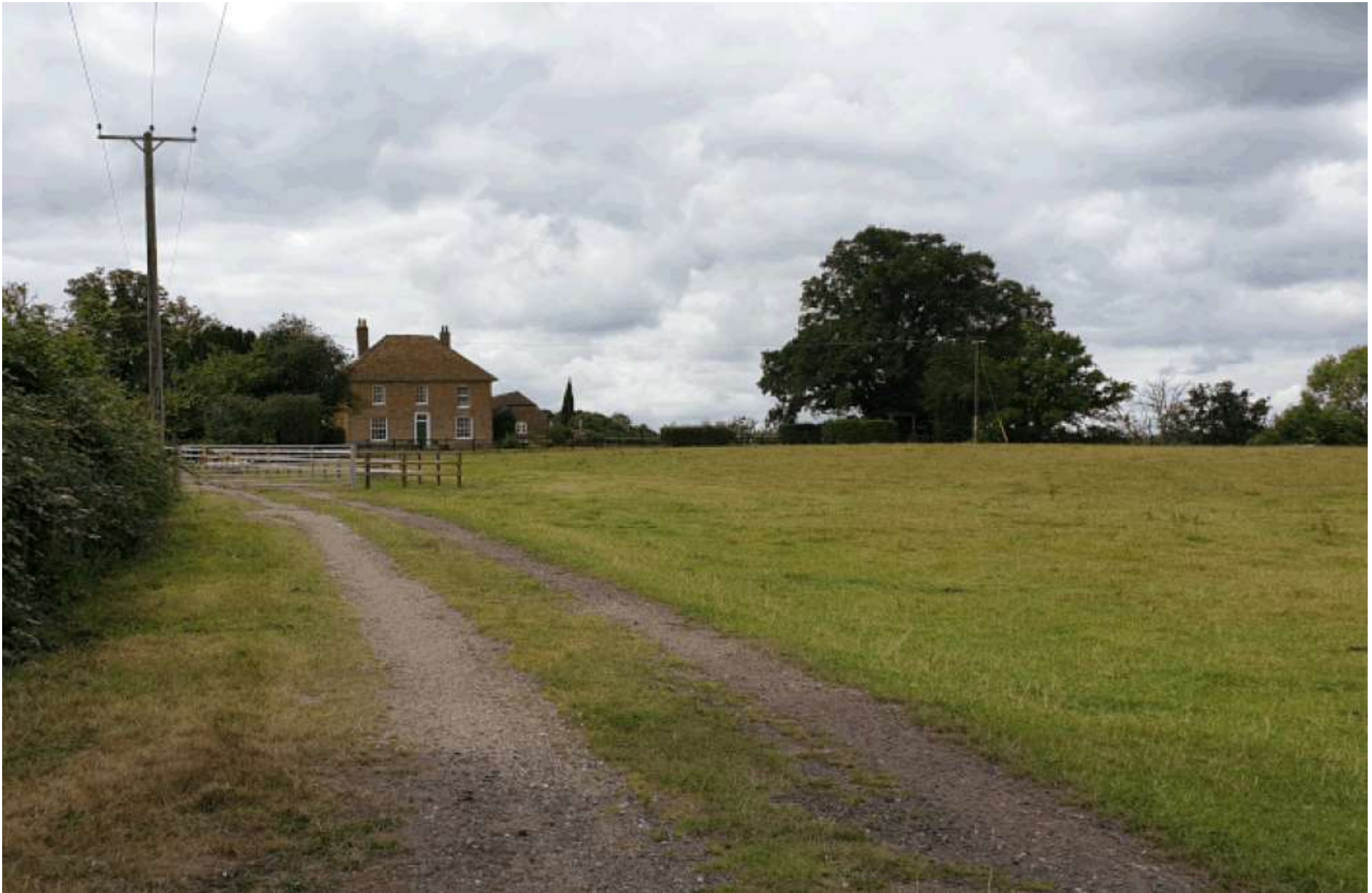
View of Grade II Listed Boames Farmhouse (looking west)
